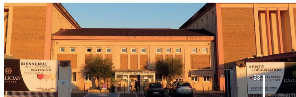
Gallician cooperative wine storehouse
